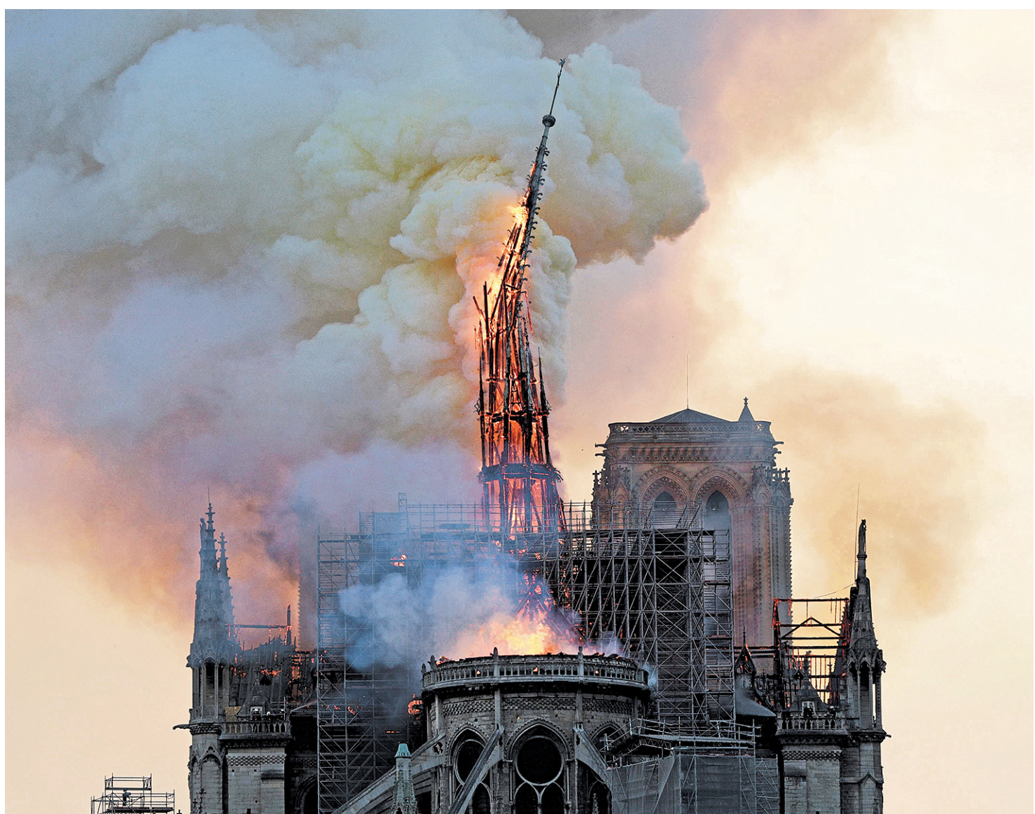
The spire of the landmark Notre-Dame cathedral in Paris collapsed on Monday as a fire raged in the medieval Gothic structure.
