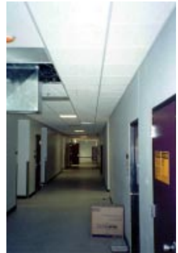
MEB hallway (after)
